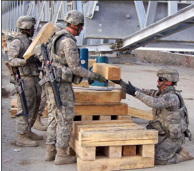
SOLDIERS from the 27th Engineer Battalion (Combat), Fort Bragg, NC, a part of the 372nd Engineer Brigade's downtrace in Afghanistan, work on constructing footers during the building of the Saracha Bridge in Nangahar Province, Afghanistan.
